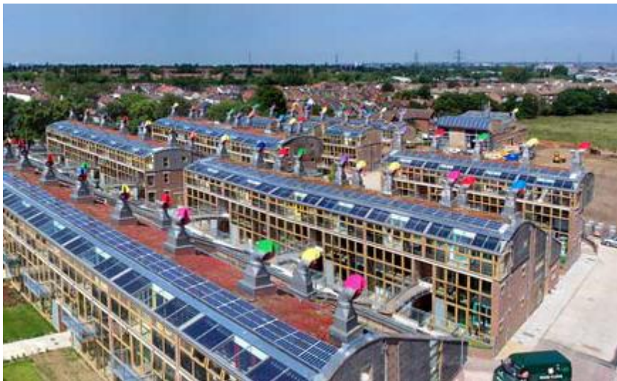
Londra – Quartiere BedZED - Beddington Zero Energy Development
